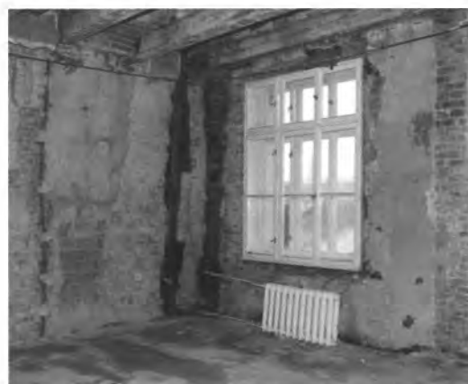
Third floor rooms from the backyard side (January 2001)
