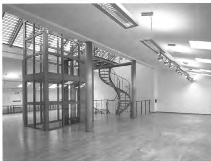
Rooms of the 4th floor with the steel-glass lift construction (June 2001)
