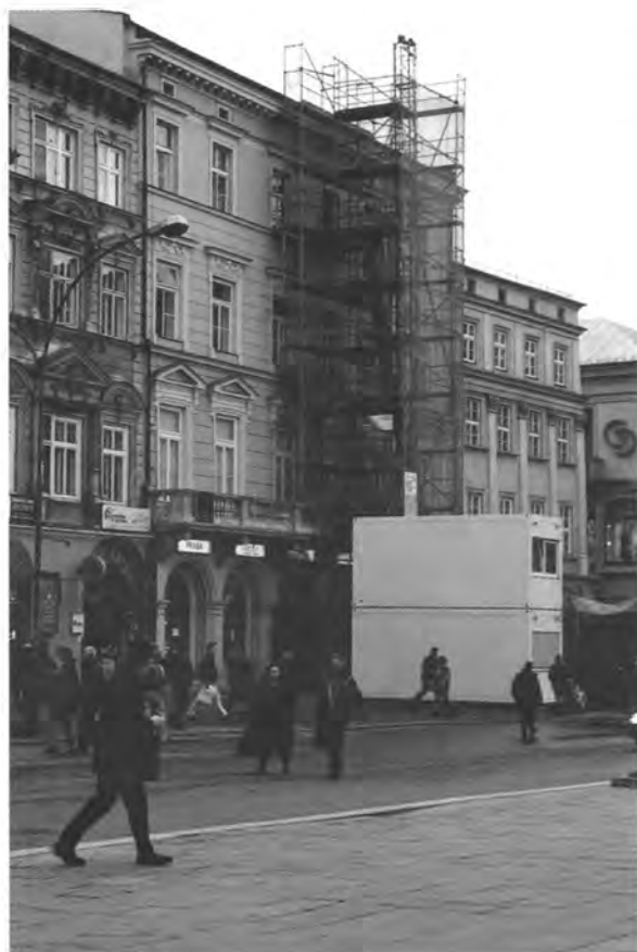
Front façade during the renovation (December 2000)
