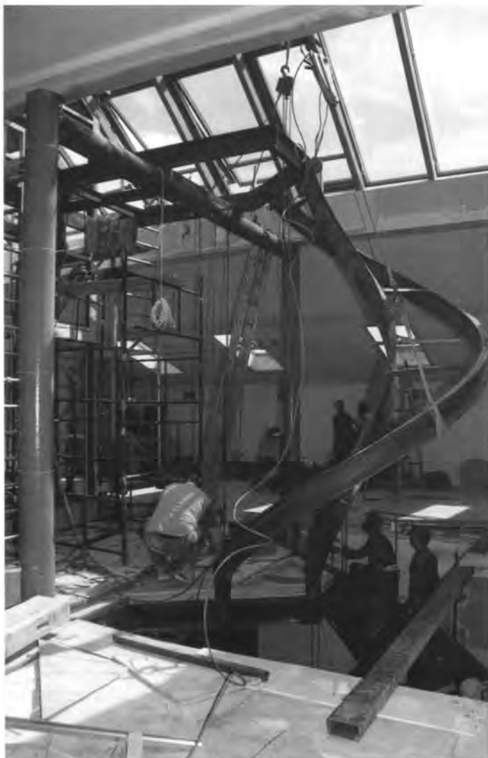
Assembly of the winding stairs leading to the 4th floor and the scenic bridge (May 2001)
