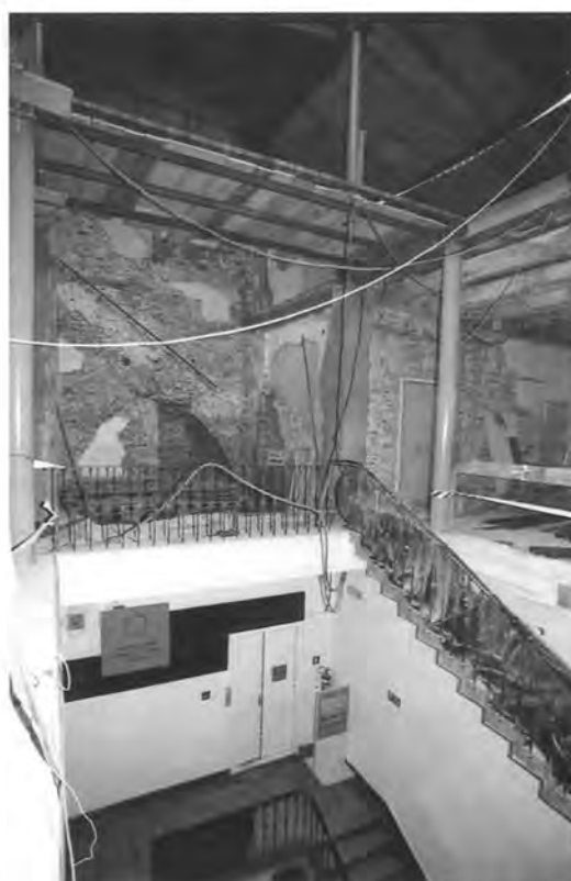
The staircase (January 2001)
