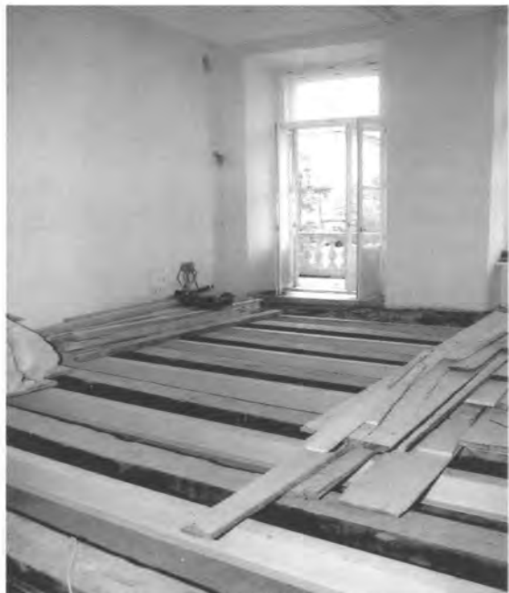
The ICC Gallery undergoing further renovation works
