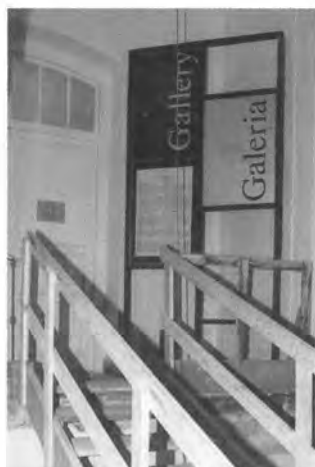
This was once the way to enter the Gallery... Conversion of the staircase allowed to install the lift for the handicapped according to the design by Atelier Loegler i Partnerzy Sp. z o.o. (February 2001)
