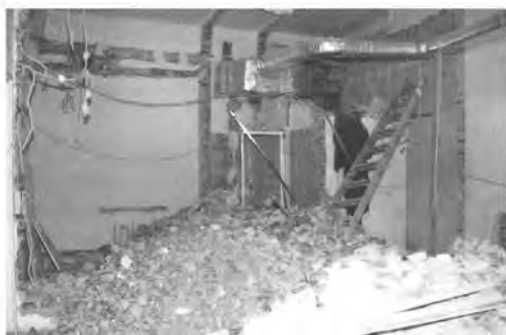
Former back of the Gallery being adapted; works with ventilation shafts (July 2003)
