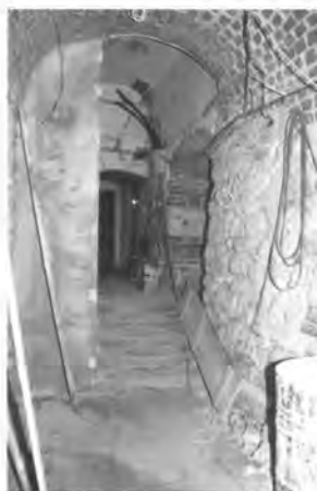
Floor levelling works in the central room (February 2003)
