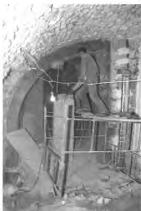
Knocking down the concrete pillar in the main room of the cellar (February 2003)
