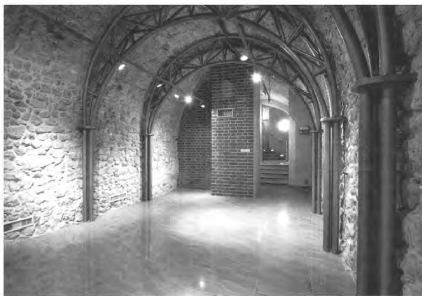
Main room with the grid support of the ceiling (May 2003)
