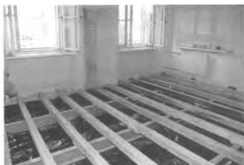
Reinforcing the ceilings over the 1st floor
