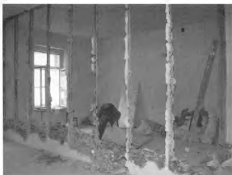
One of the partition walls is being demolished
