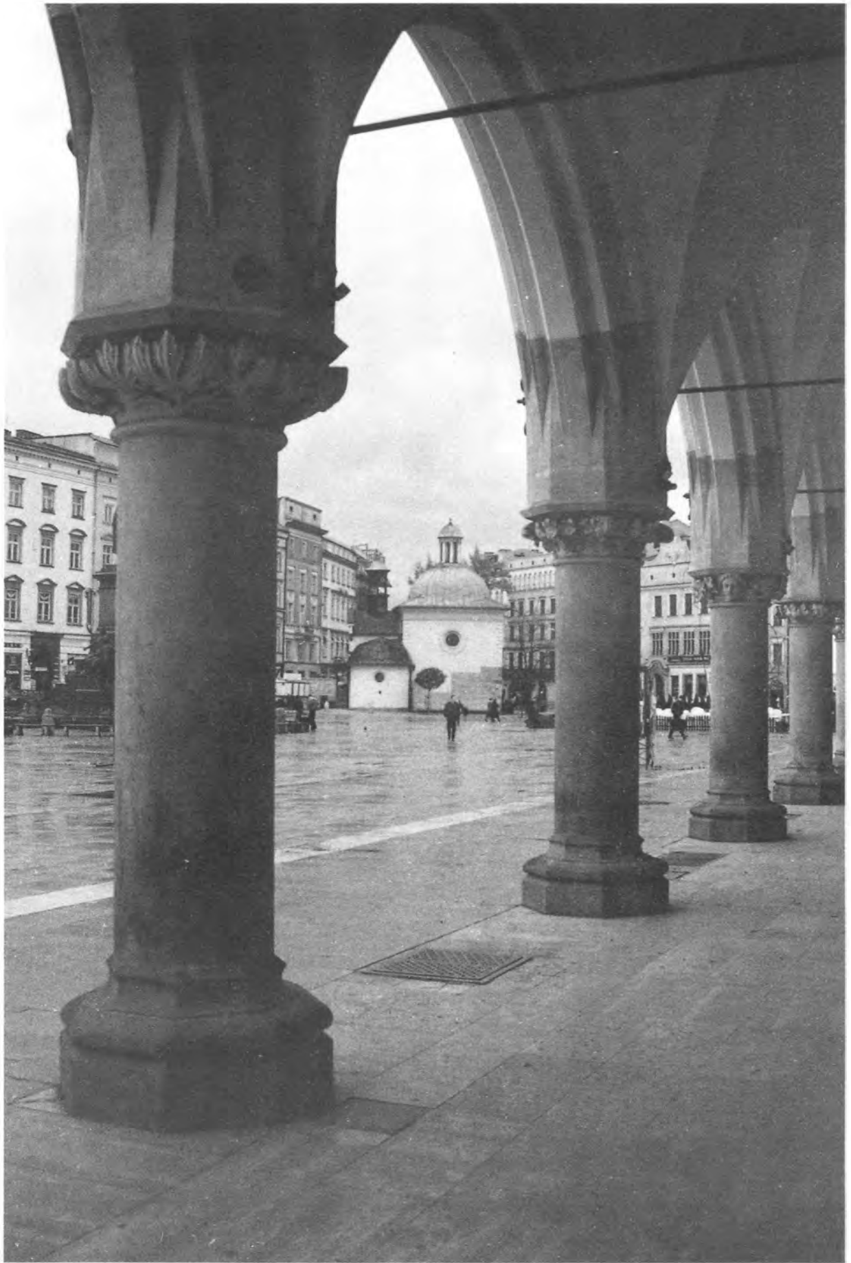
20. Arcades of the Cloth Hall with a view of St Adalbert's Church on the Market Square
