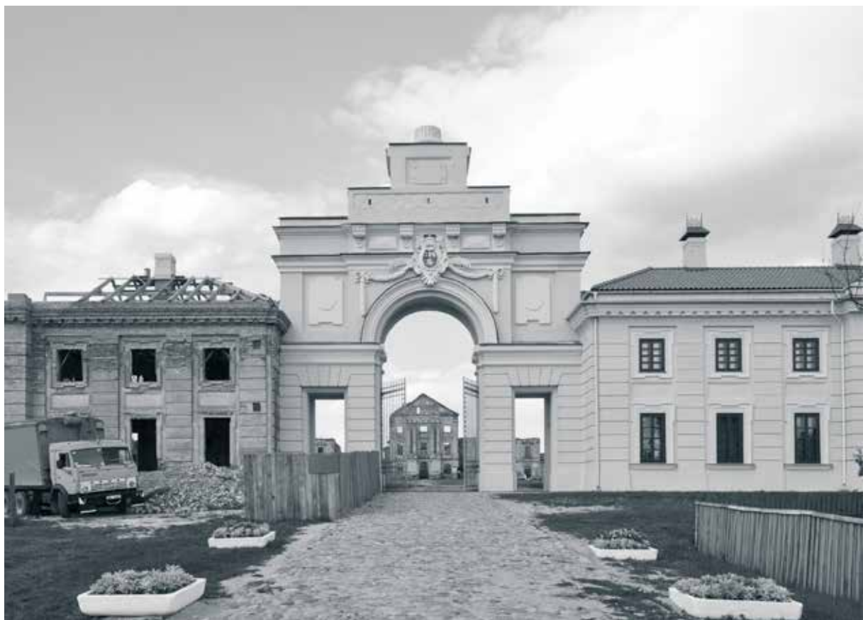
Renovation of the main gate of Sapieha Palace in Ruzhany
