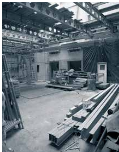
The Ravens Hall – new steel ceiling beams (February)
