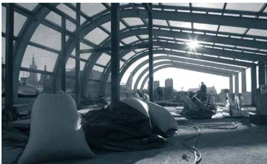
Annexe building – glazed panoramic room (March)
