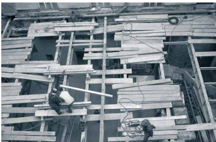
Patio – a new ceiling of the Ravens Hall, i.e. the patio floor, will soon be ready (February)
