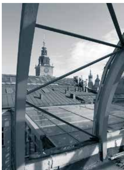
Annexe building – wall truss of the panoramic room (February)
