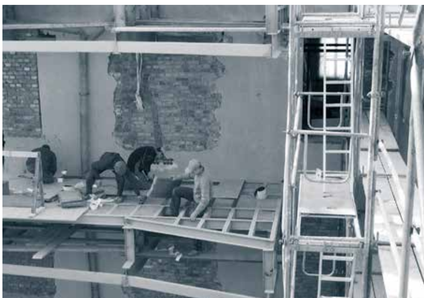
Patio – the structure of the bay window is built for the future Roland Berger Reading Hall (March)
