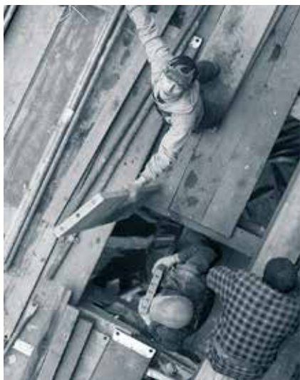
Patio – working without heavy building machines required enormous organisational skills (January)
