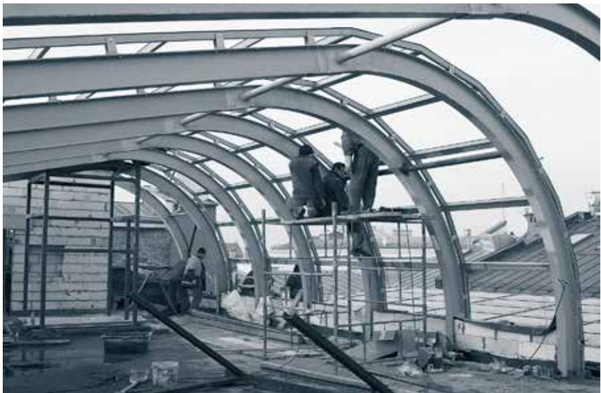
Annexe building – installation of the framing of the glass wall and roof panels for the panoramic room (January)
