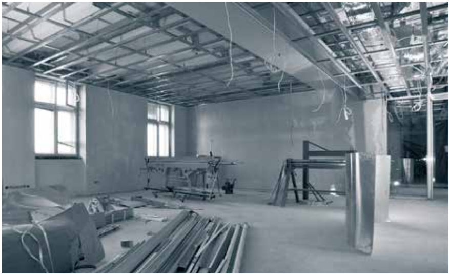
Annexe building – finishing works in the new ICC Library (August)
