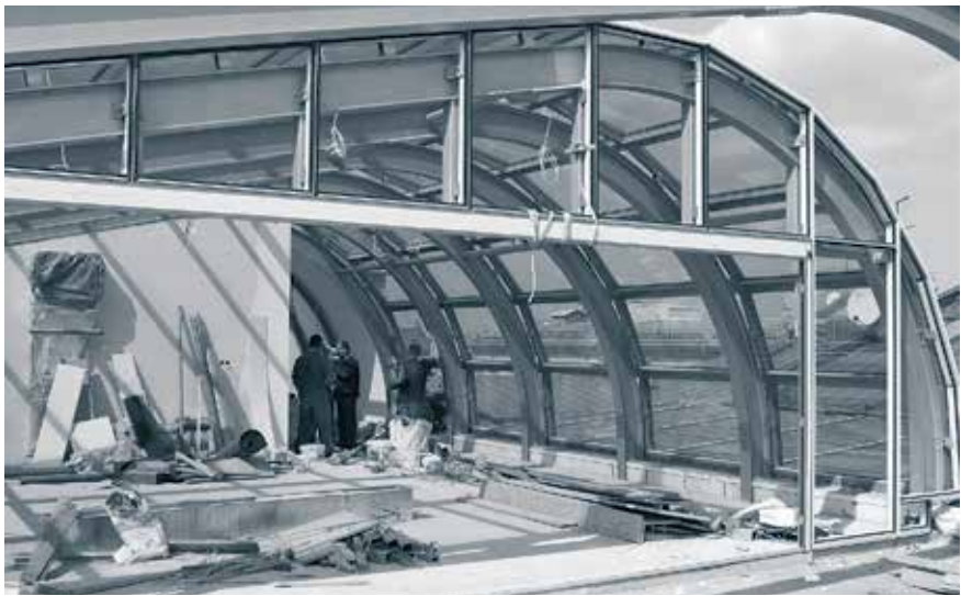
Annexe building – finishing works in the panoramic room (September)
