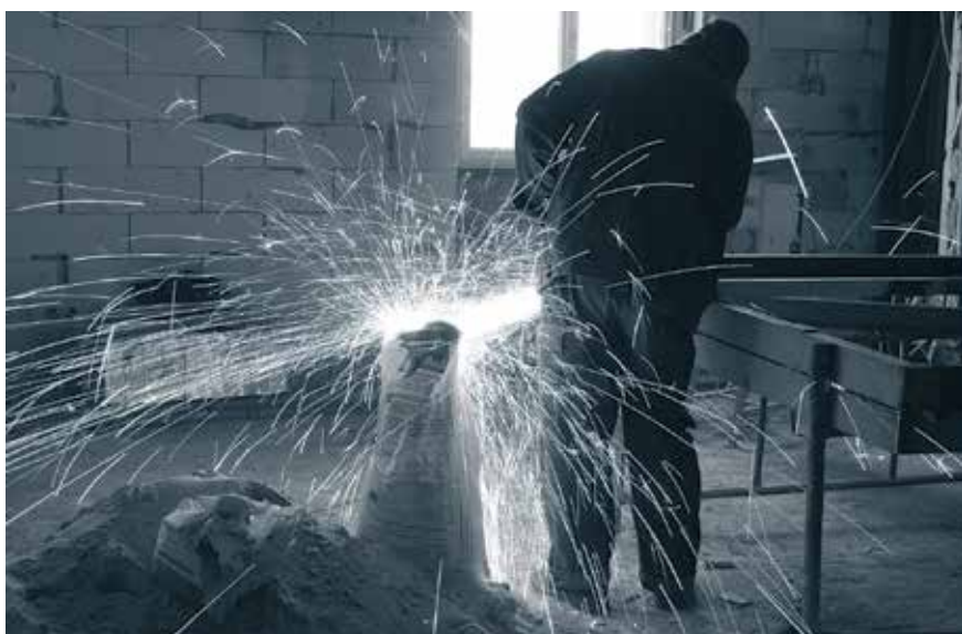
Annexe building – a number of the steel elements were made on the spot (March)
