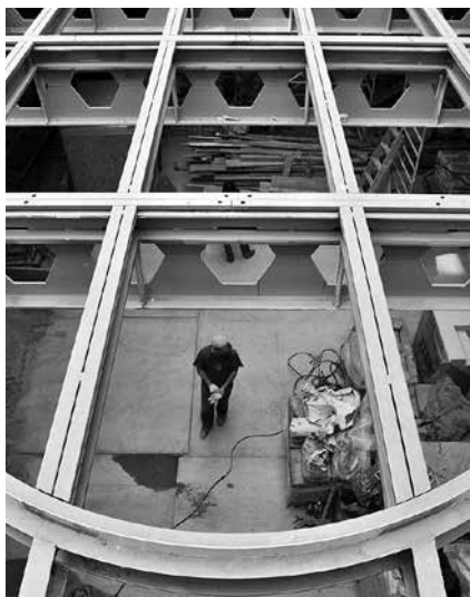
Patio – skylight of the Ravens Hall in the making (April)
