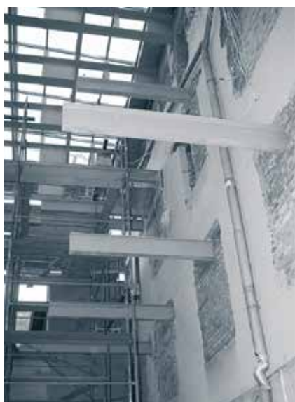
Patio – steel supports for the bay window of the future Roland Berger Reading Hall (February)
