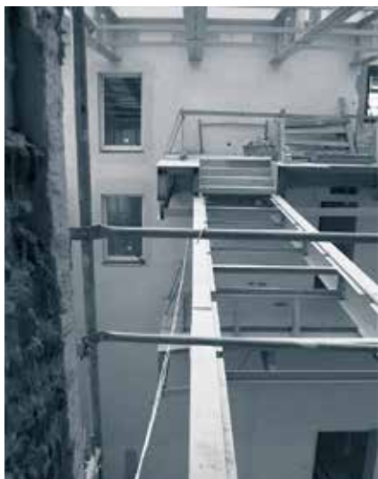
Patio – building a bridge between the front building and the annexe building (May)
