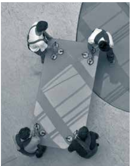
The Ravens Hall – glazing the skylight (June)
