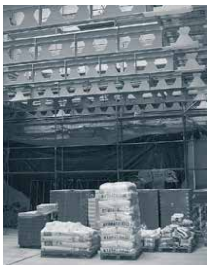
The Ravens Hall – steel beams of the new ceiling (April)
