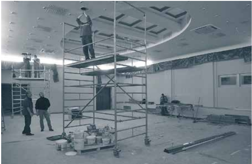
The Ravens Hall – finishing works (December)
