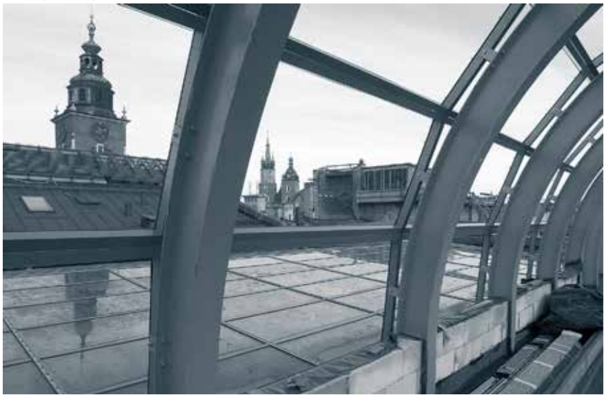
Annexe building – framing of the glass wall and roof panels for the panoramic room (January)
