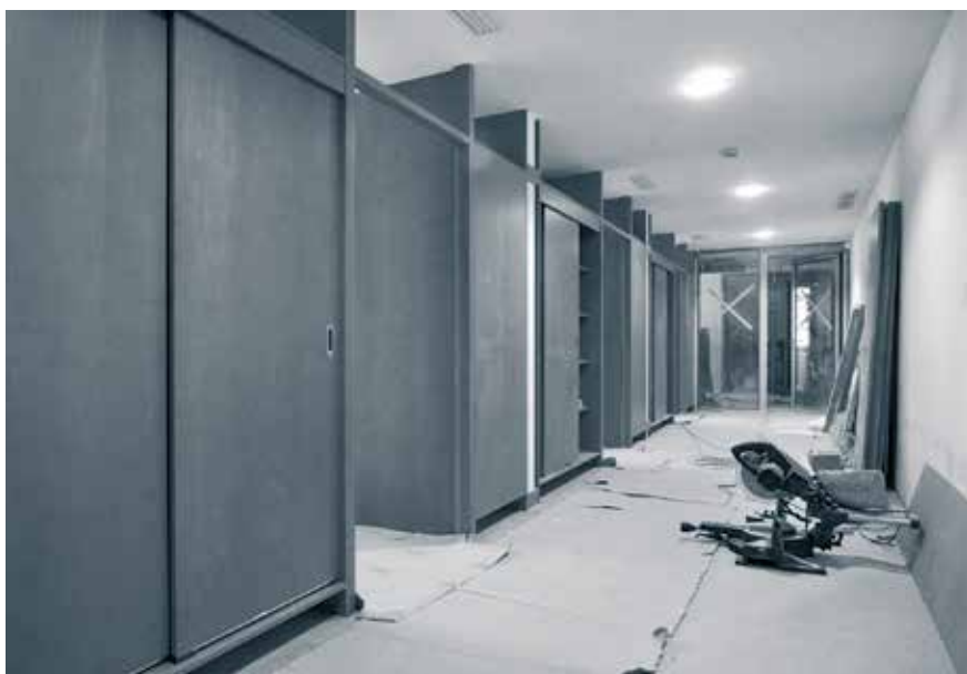
Annexe building – finishing works in the administrative rooms of the ICC (November)
