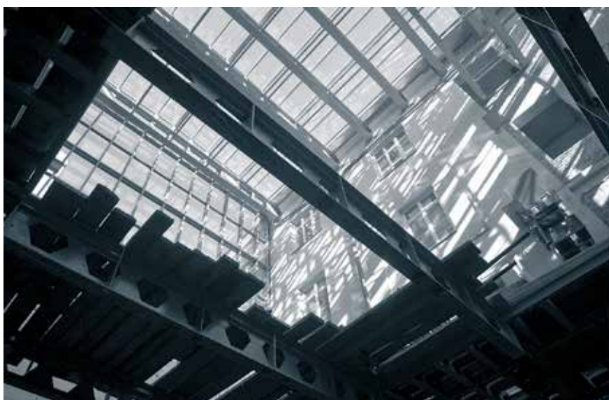
The Ravens Hall – a new skylight will be put here (February)
