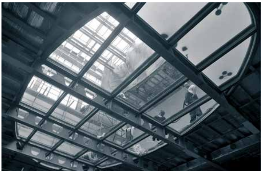
The Ravens Hall – glazing the skylight (June)
