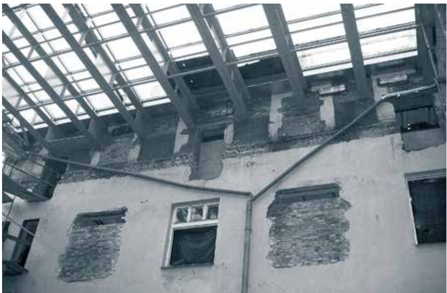
Patio – the beginning of indoor works (January)
