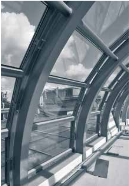
Annexe building – glazing the panoramic room (September)
