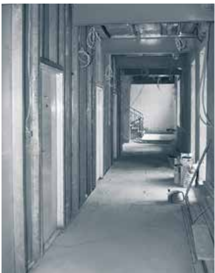
Annexe building – partition walls in the new rooms of the European Heritage Institute (April)
