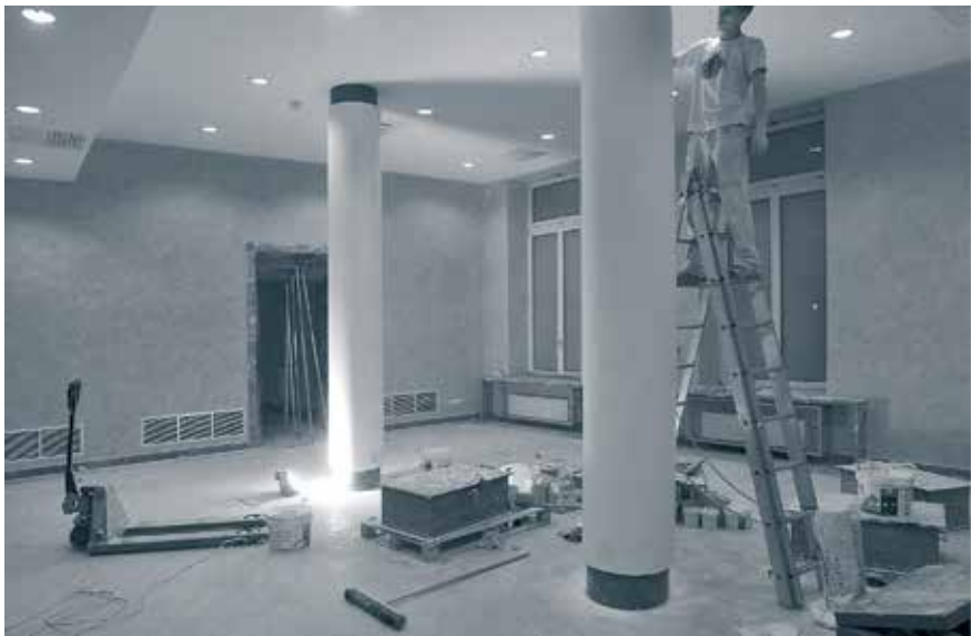
Annexe building – finishing works in the foyer of the Ravens Hall (December)
