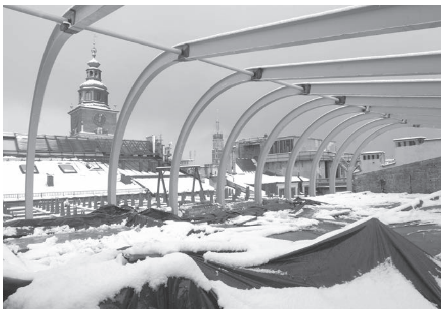
November – insertion of girders for the glass roof over the ICC courtyard and fins supporting the transparent roof of the annexe
