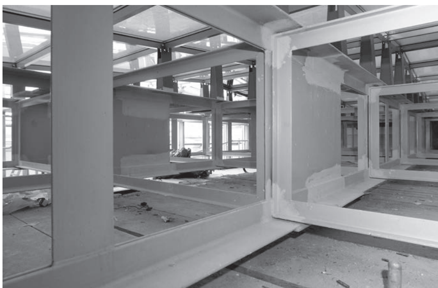
December – insertion of the panels into the glass roof and the curtain walls of the ICC courtyard commences
